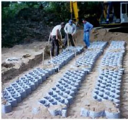
3. FIELD OR FILTER LAYOUT SPACING AS PER DESIGN
